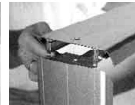
A close up of the final E-Z Frame section being fit into place. ABC's Corner Key system makes assembling small sign cabinets a snap! Suitable for indoor applications and small outdoor signs.
