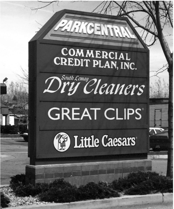
Monument sign with routed push-though lettering and flush copy panes.
